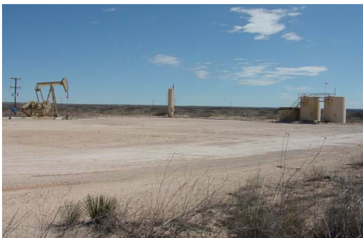
Figure 50. Typical oil well pad and associated structures with an overall footprint of the pad approximately 1-2 acres in size (Photo courtesy of NMDGF).
