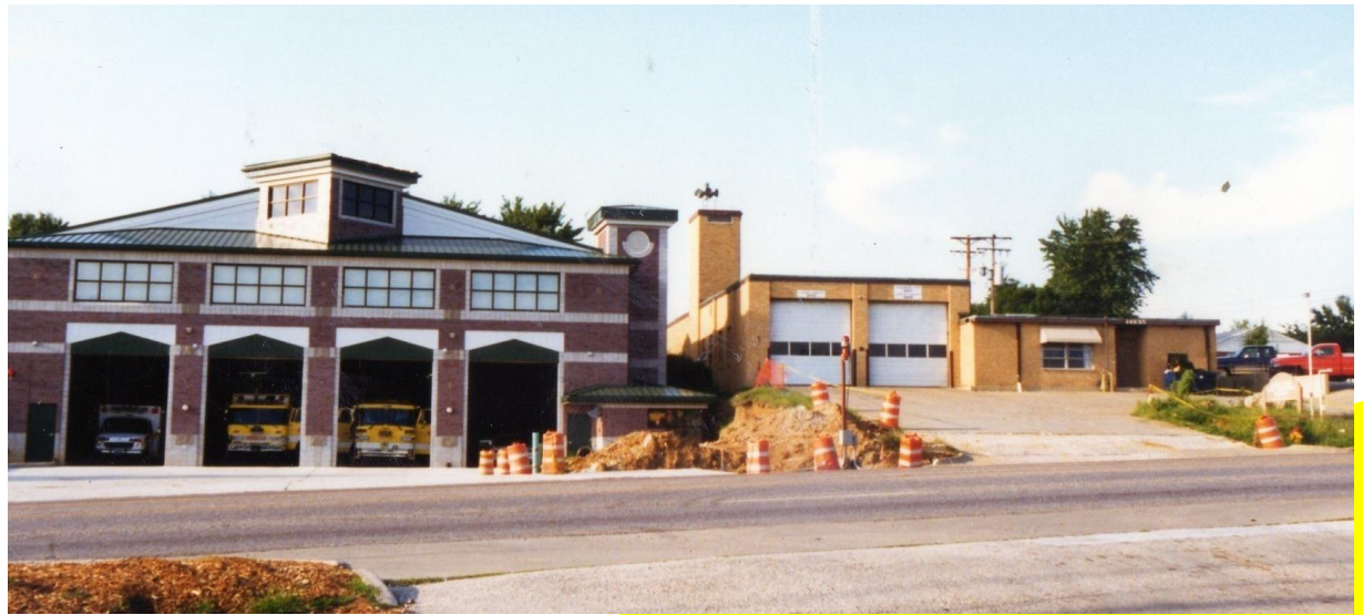
Station #1 - Ballwin addition 1966 Current Station 1996
