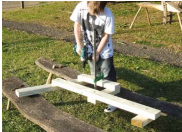
Stage 2: Fix the first part of the platform.
