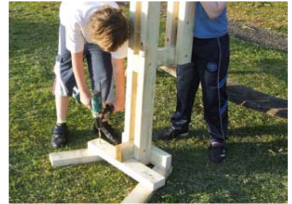
Stage 6: Fix the rear leg brace to the rear legs.
