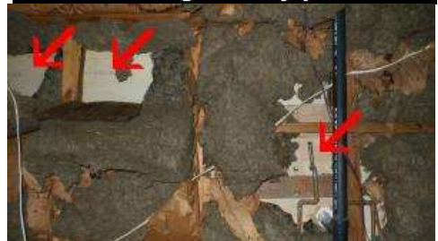
insulation is generally poor
