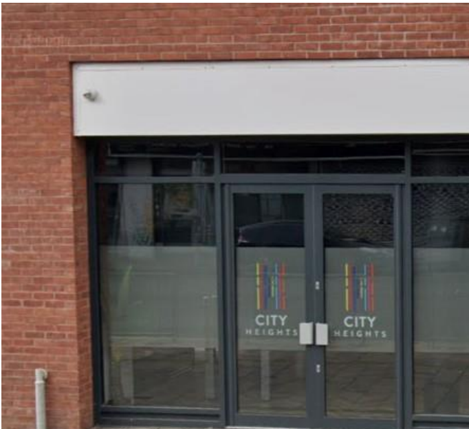
Proposed (primary) materials - brick and render with large format 'punched hole' fenestration and shopfronts
