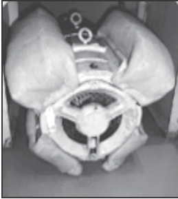
New Clean Installation Imperial 366
