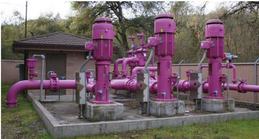
Figure 5.2. “Purple pipes” in Sonoma County, California, deliver recycled water for irrigation uses (Sonoma County Water Agency)
