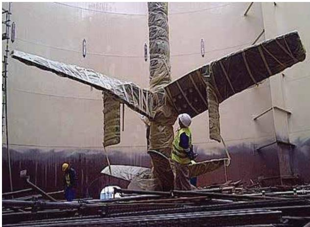
Mixtec has successfully designed and commissioned mechanical agitators to operate in tanks larger than 6000 cubic meters, with agitator systems in excess of more than 38 tonnes, impellers manufactured over 7.6 meters in diameter and with shaft lengths of over 21 meters. For such applications, Mixtec's Series 4000 heavy-duty agitator drives are available in standard models up to 450 kW but can easily be upgraded to suit the application.
