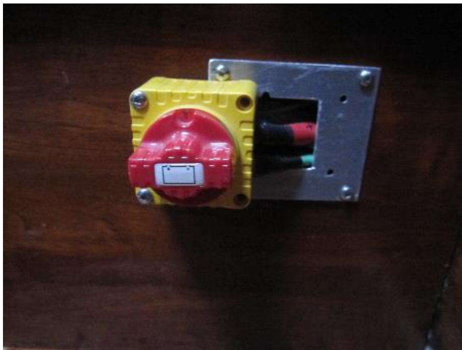
Figure 107 Battery Disconnects
