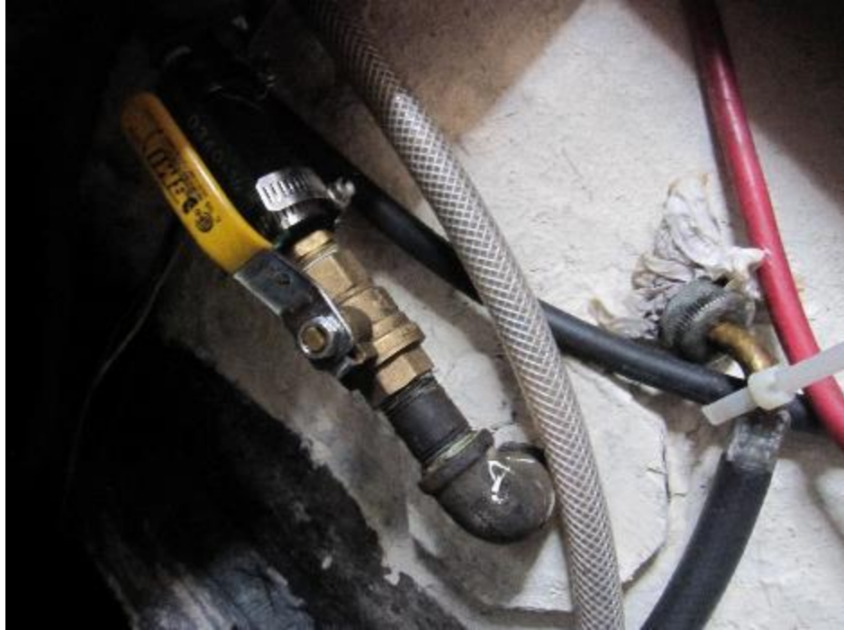
Figure 114 Through Hull
