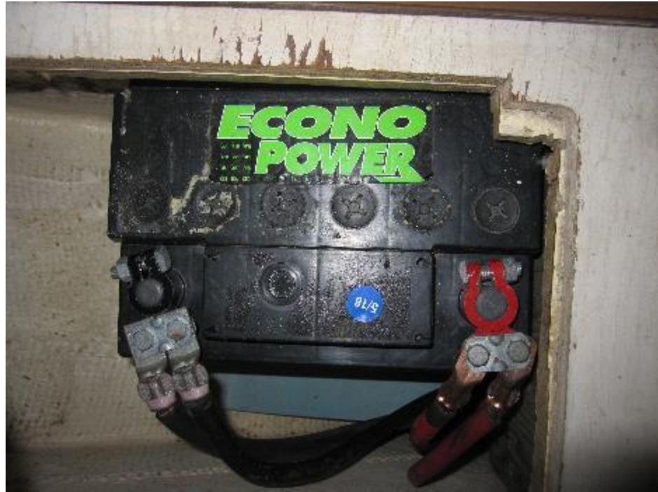
Figure 103 Starting Battery
