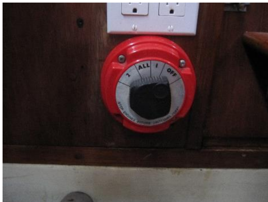
Figure 106 Battery Disconnects
