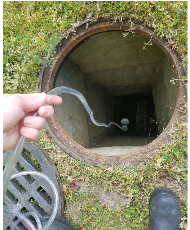
Lowering the inflow tube down into a storm drain; the bottom of this pipe is about 12 feet from the ground surface
