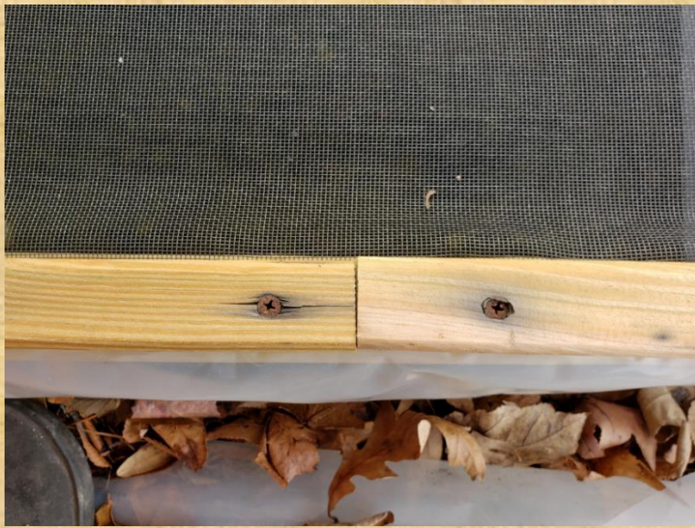
8ft 1x2 with added 2ft section to make 10ft piece. Screws were backed out one side at a time
