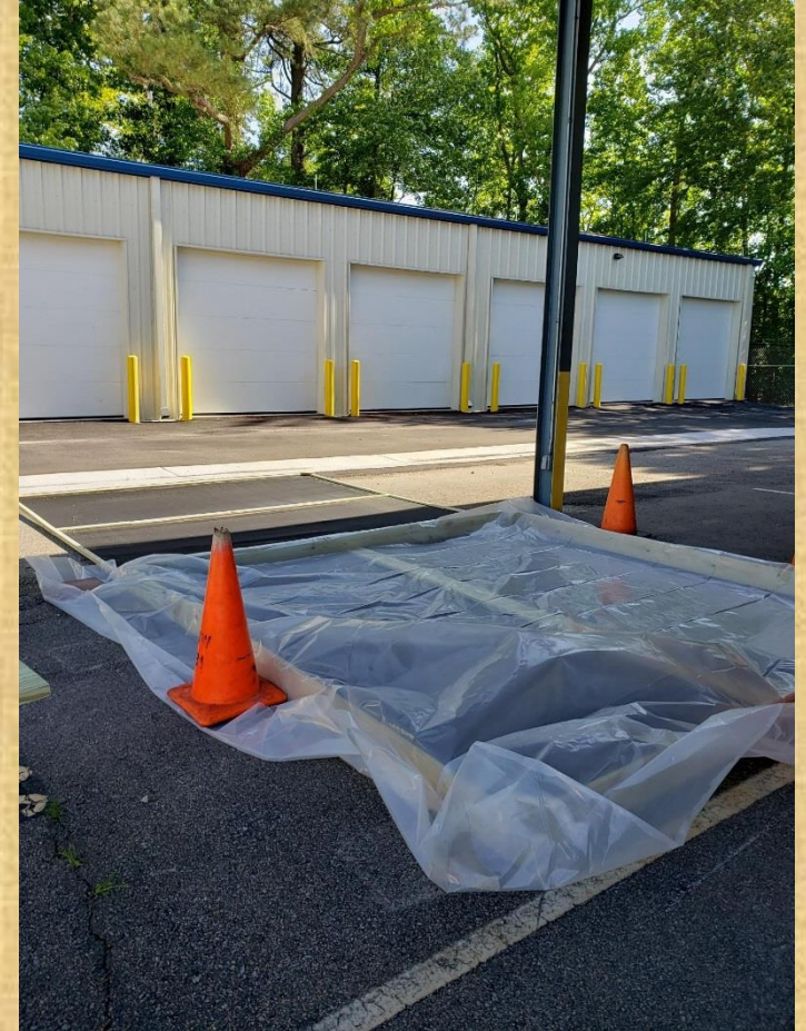
Plastic laid inside ready for water
