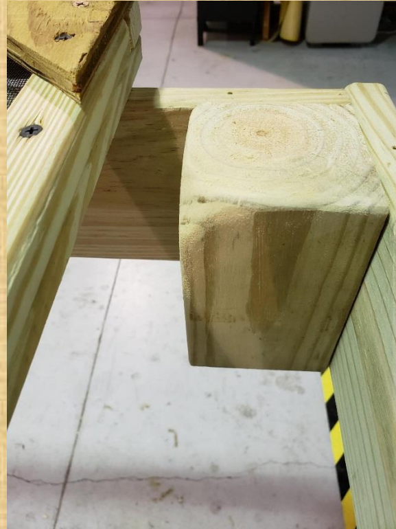
Smooth edge to protect liner
