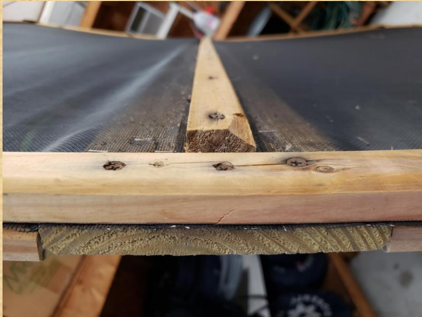
Top frame support beam (used 1x6- 10ft )
