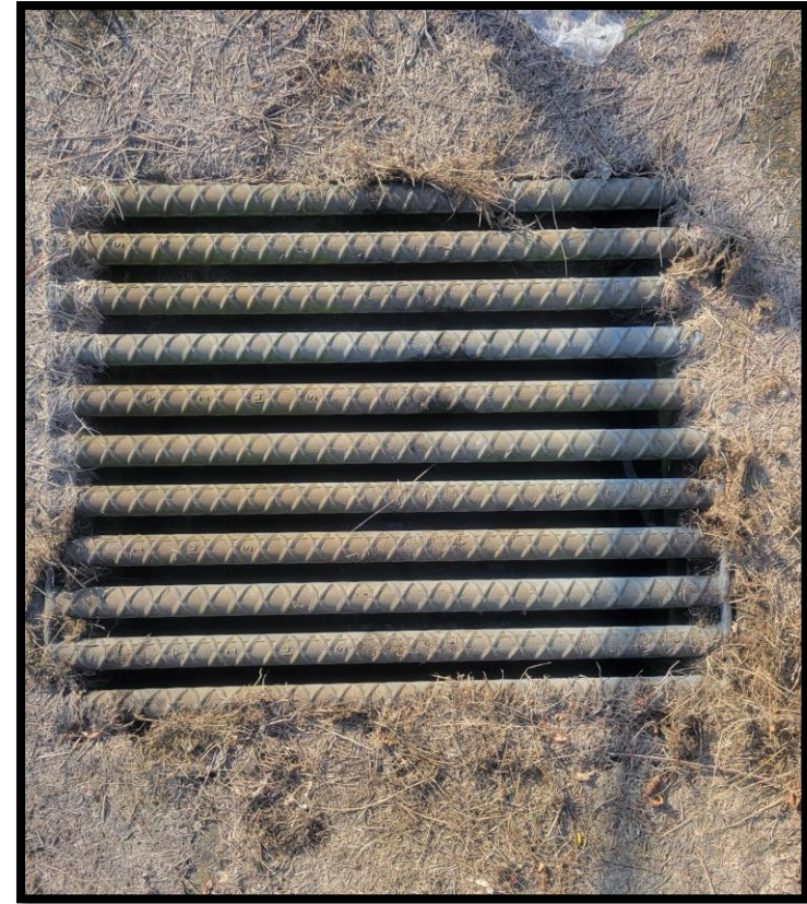
Drain next to pump station holding water
