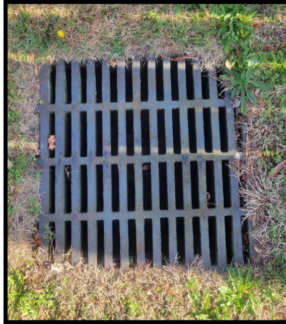
Grate holding water next to P.S.
