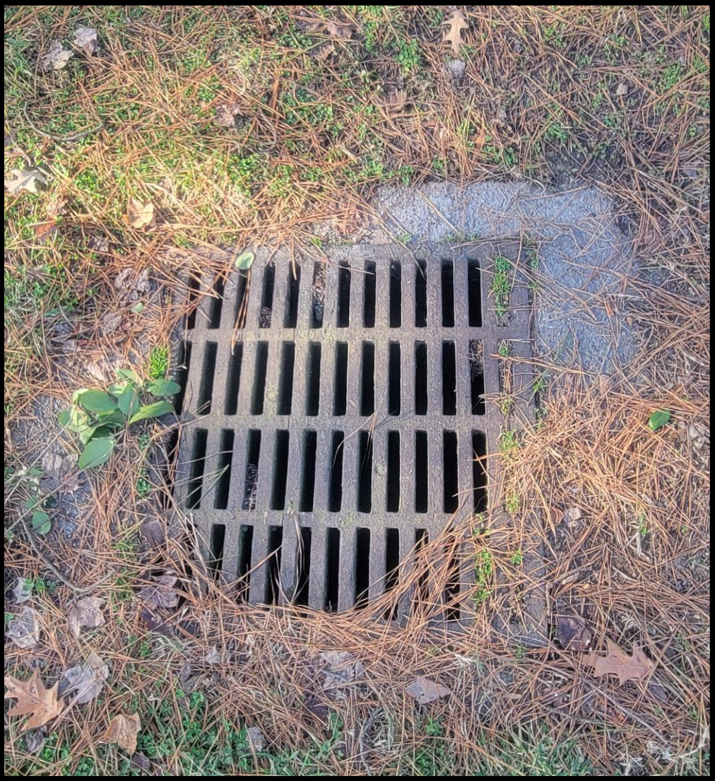
Older neighborhood- drainage system of driveway pipes, swales and grates
