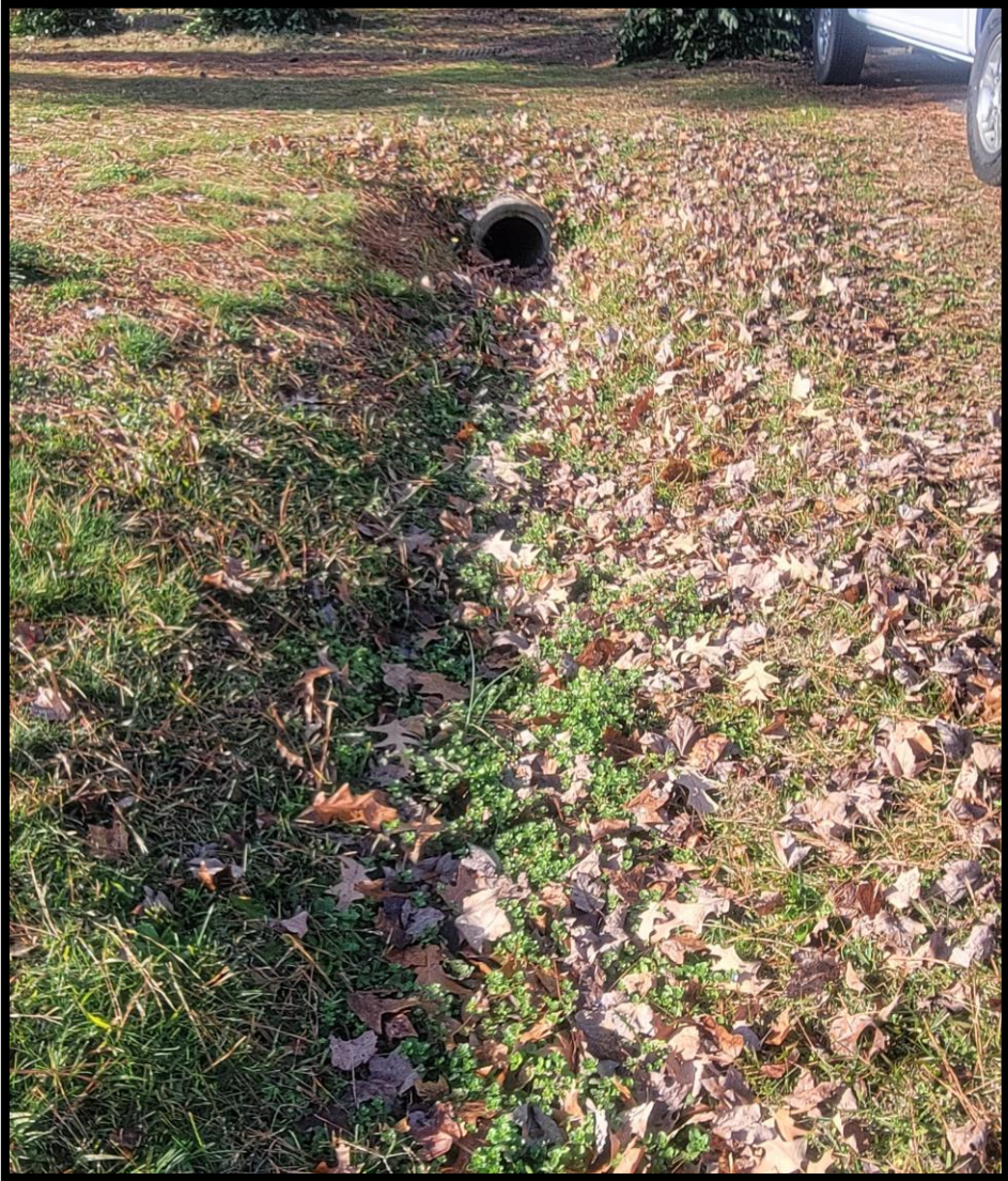
Older neighborhood- drainage system of driveway pipes, swales and grates
