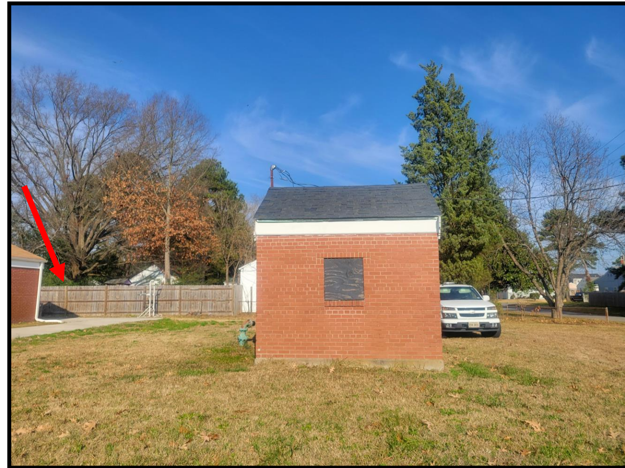
Older neighborhood with broken down CDI system
