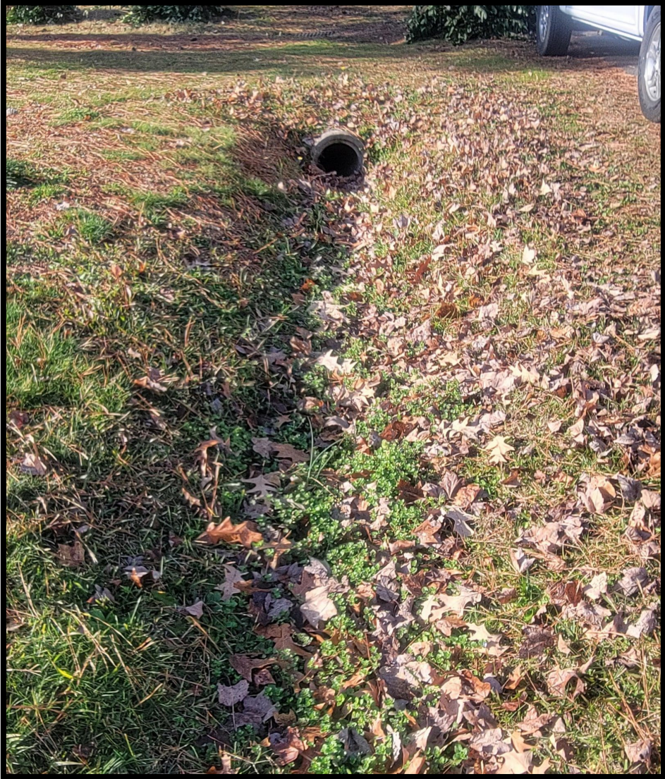
Non-pumping station site. Older neighborhood- drainage system of driveway pipes, swales and grates
