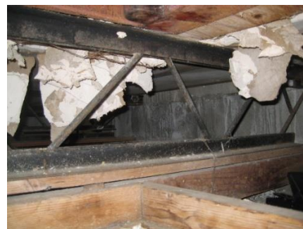
Attic space near hatch.
