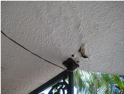
Rebar in breezeway ceiling.
