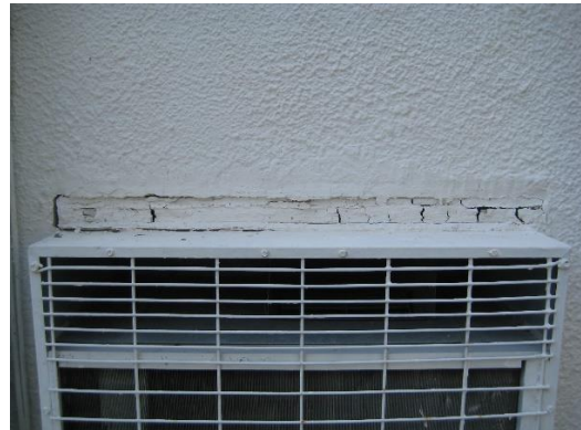
Openings around an air conditioner unit.
