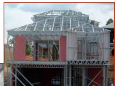
Steel frame construction
