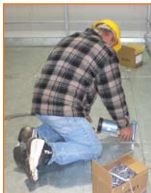
Steel floor fastening
