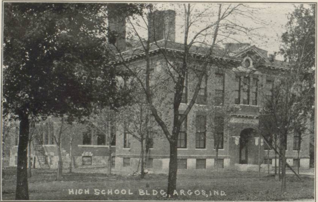
ARGOS PUBLIC SCHOOL BUILDING
