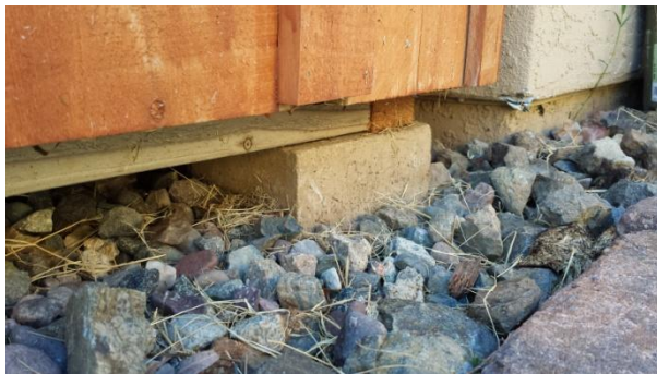
FIGURE 21: STRUCTURE AND FRAME SUSPENDED ON CINDER BLOCK
