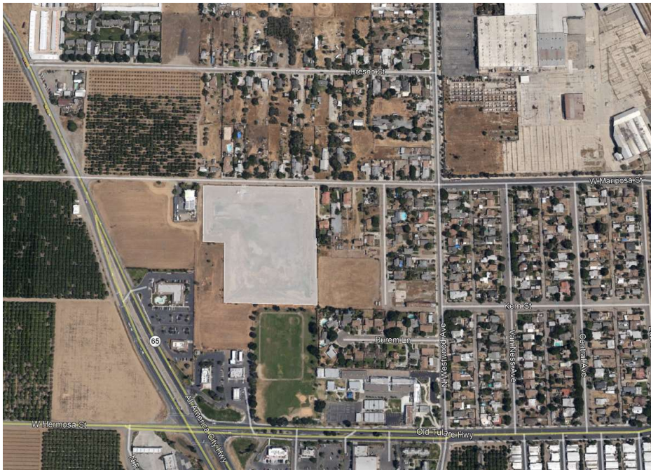
Figure 5-7 City of Lindsay Recharge Basin Site
