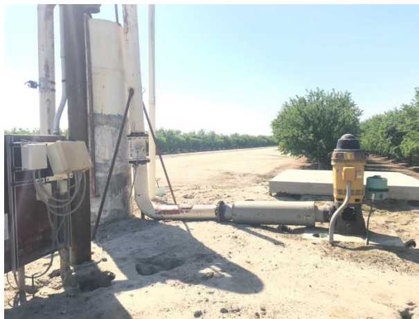
Figure 1 - Meter installed 2.5 diameters downstream of a 90° bend
