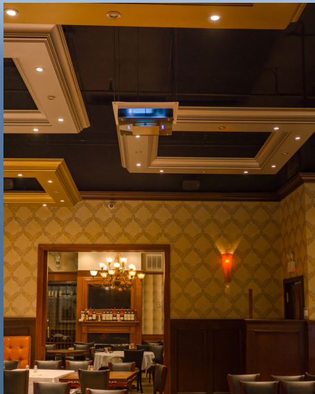
Zone360 installed at Rocco Steakhouse
