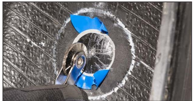
**17.** With the blue poly still positioned under the cap, stitch the repair unit from the center out using firm pressure.
