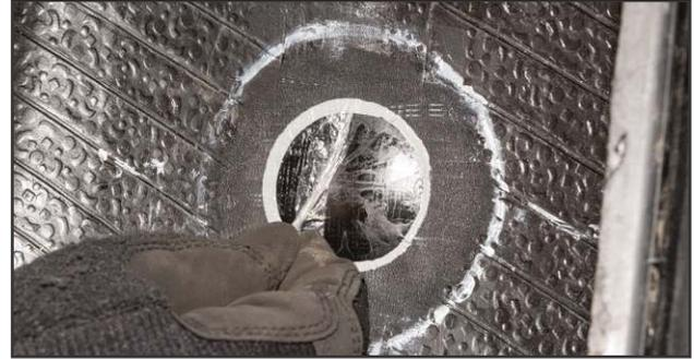
**19.** Remove the clear protective poly from the top of the repair.
