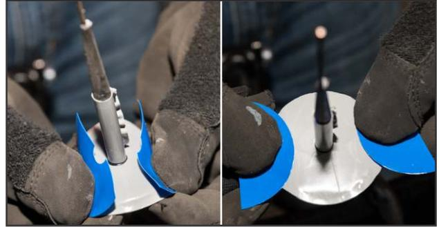
**13.** Reposition the poly on the cap to prevent contamination of the gray gum and allow easier removal of trapped air during installation.
