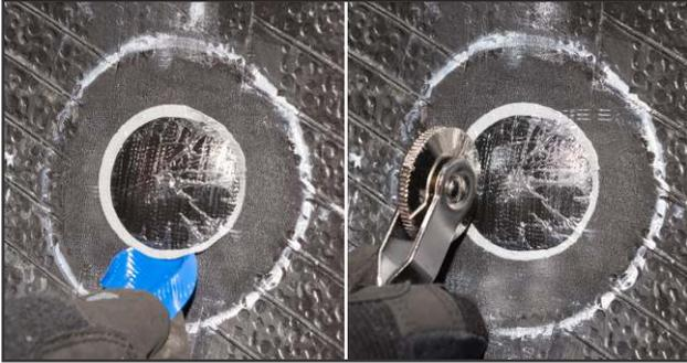
**18.** Remove the poly from the cap, press down the sides and continue stitching toward the edges of the repair. Stitch with firm pressure in the opposite direction to ensure air is removed.
