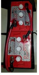
Batteries banks located below seating area in accommodation, no proper ventilation applies to batteries storage area.
