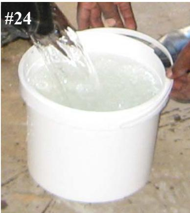
24. Small bucket for measuring water, sand and gravel when making concrete.
