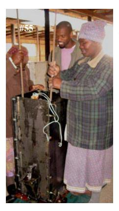
55. Steel rods approximately 16 mm in diameter and 1.5 meters long for working concrete.
