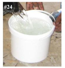
24. Small bucket for measuring water, sand and gravel when making concrete.
