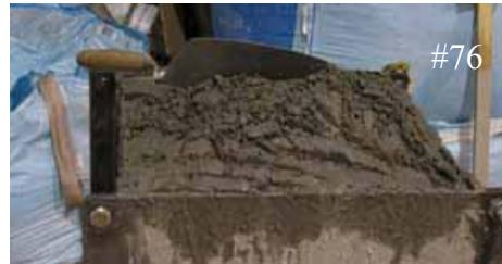
76. Wood wedge is removed. Surface is 'chopped' up using a trowel
