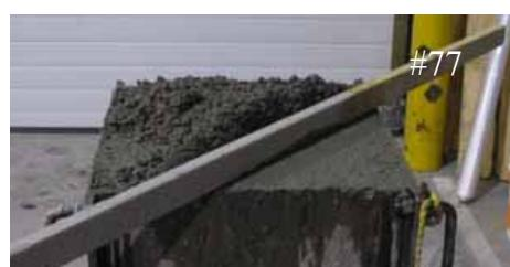
77. A straight piece of wood is used to level the surface (also called 'floating').
