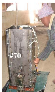
69. **Rodding** the concrete using a steel rod. (Insures that concrete is in all places. Be careful not to disturb standpipe.)
