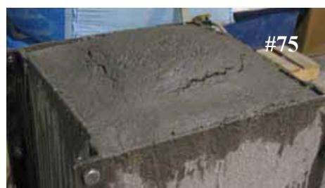
74. Concrete, with wood wedge in place is allowed to 'set' for 3 to 4 hours.
