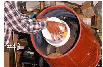
Mixture is well mixed before water is added. Start with one measure of water. Mix well. Keep adding measures of water until it looks 'close' – on the verge of looking 'runny'.
