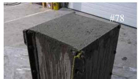
79. Mold is cleaned up and concrete is allowed to set for another 18 to 24 hours.
