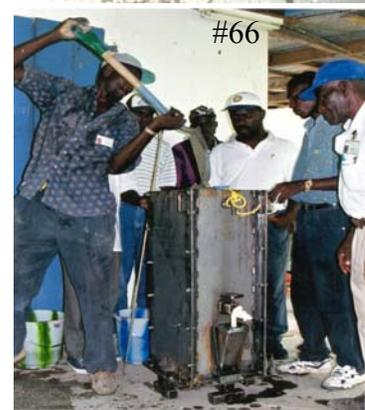
66. Adding concrete to mold.
