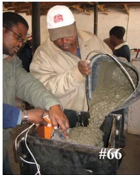
67 – 68. Adding concrete to mold.
