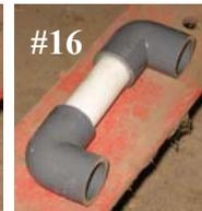
(Note that there are two systems for cementing pipe. One uses a primer and cement and the other uses a combined primer – cement. Both are good.)
