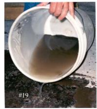
Once washed the media should be allowed to drain and dry if possible. The washed media should be stored in an area protected from contamination.
