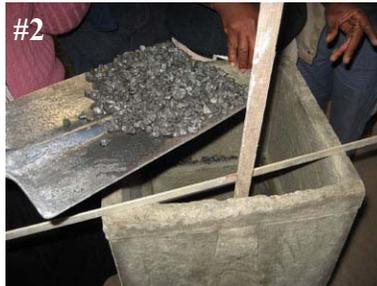
3. Leveling surface of underdrain media with hand.
