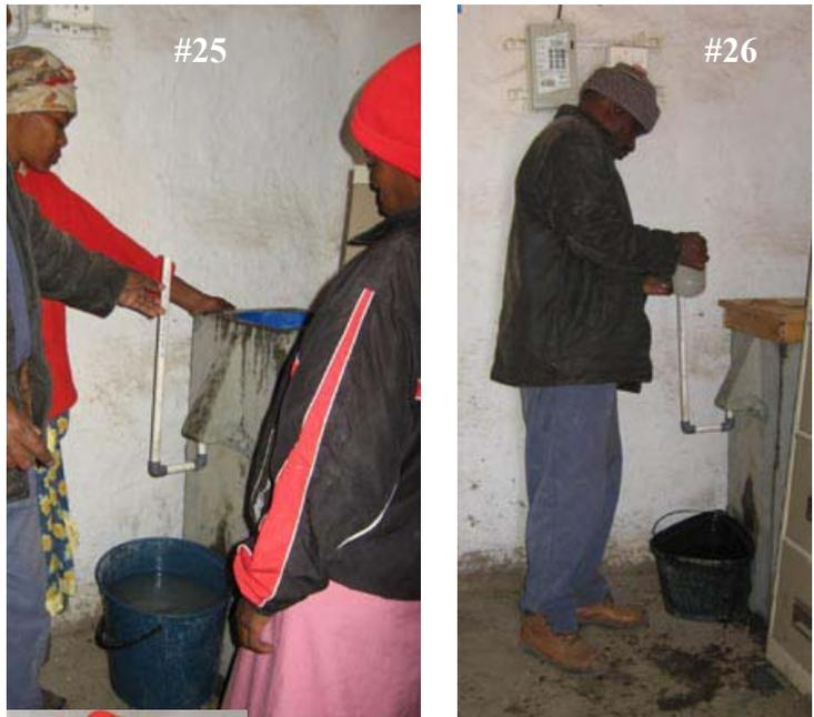
27. Pour another bucket of water into filter and allow to drain. This will flush out the chlorine solution. The filter is ready for use.
