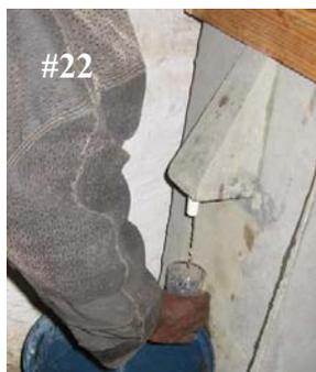
23. Initially filtered water is very cloudy (turbid) but as flushing continues water will become very clear – more clear than the source water.
