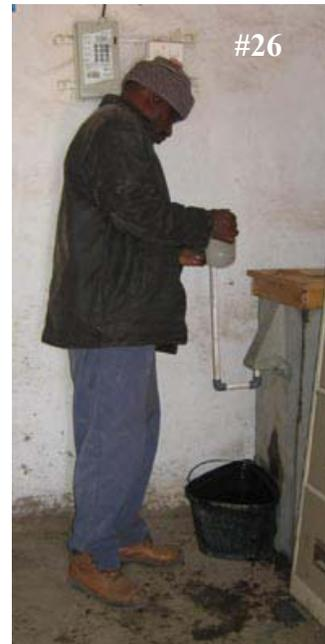
27. Pour another bucket of water into filter and allow to drain. This will flush out the chlorine solution. The filter is ready for use.
