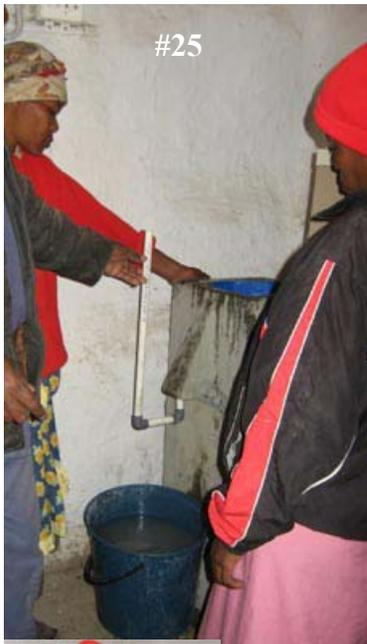
26. Pour approximately two litres of the solution prepared as described below into the top of the tube (easier if depth of water in filter is low.)
