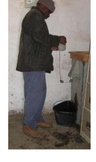
27.Pour another bucket of water into filter and allow to drain. This will flush out the chlorine solution.
