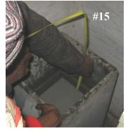
Water in filter will look very cloudy, 'dirty', or turbid during and immediately after the addition of the filter media. This is normal. The amount of turbidity will depend on the type of media used and the amount it was washed. The first step after all media is installed in the filter is to perform an initial cleaning.
