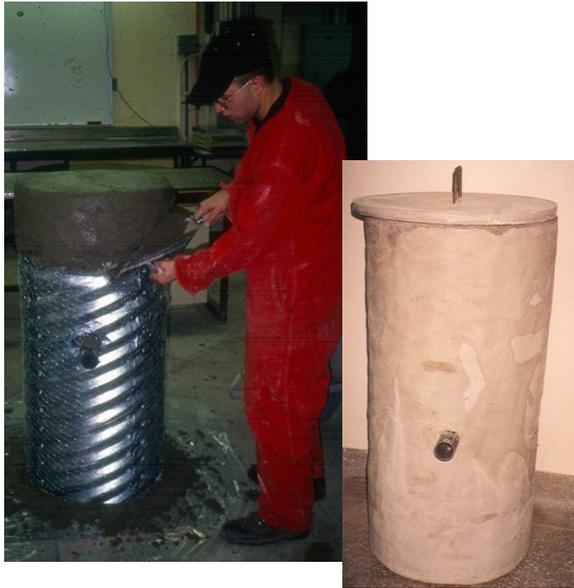
**Ferro-cement construction of BioSand Water Filter at University of Calgary.**
