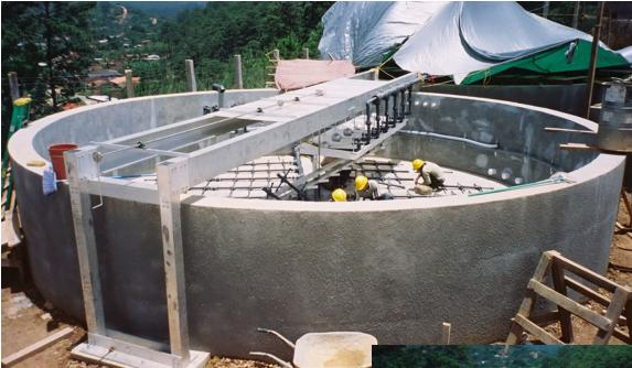
Finishing construction of the 38,000 lph BSF in Honduras.
