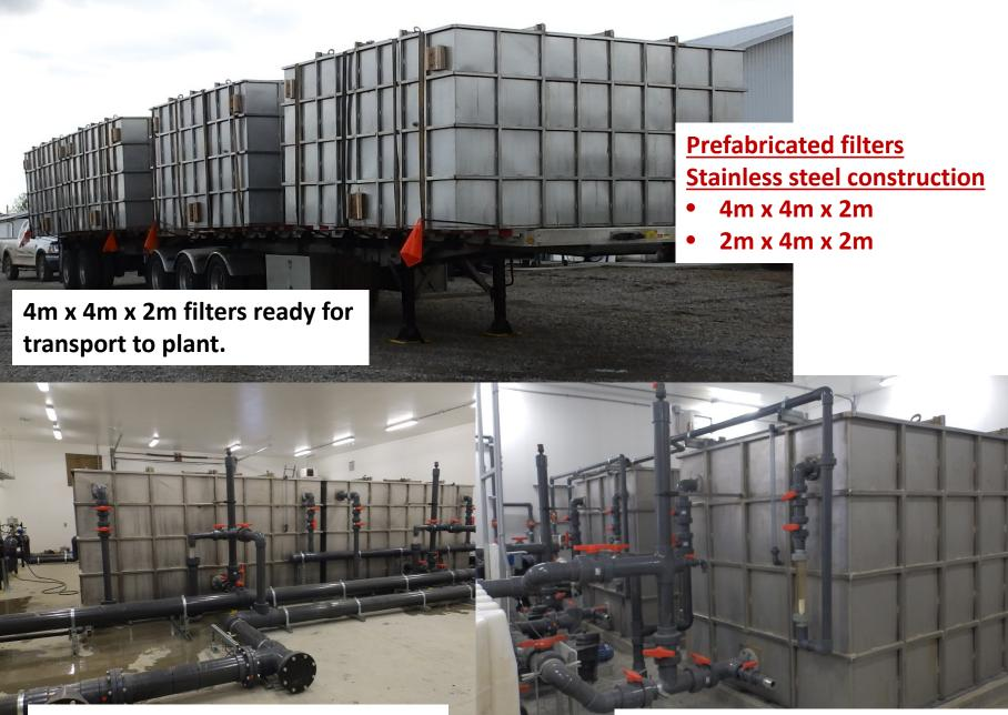
Array of four 4m x 4m x 2m filters installed and operating.
