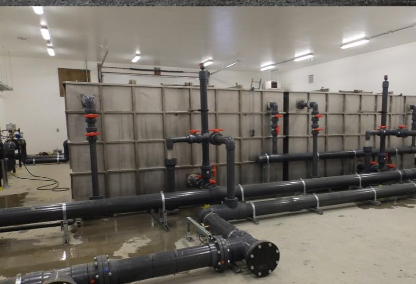
**Array of four 4m x 4m x 2m filters installed and operating.**
