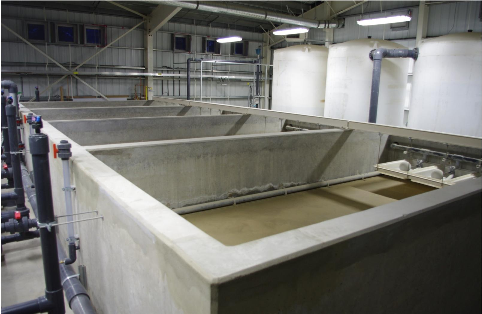
**Inside Exshaw water treatment plant showing four filters and three contact tanks.**
