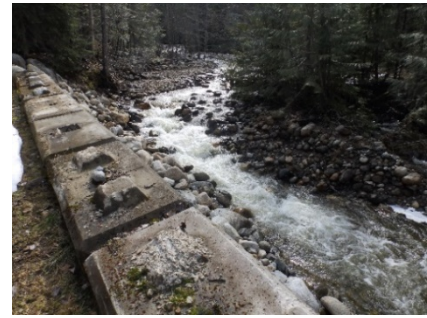
Creek water source
