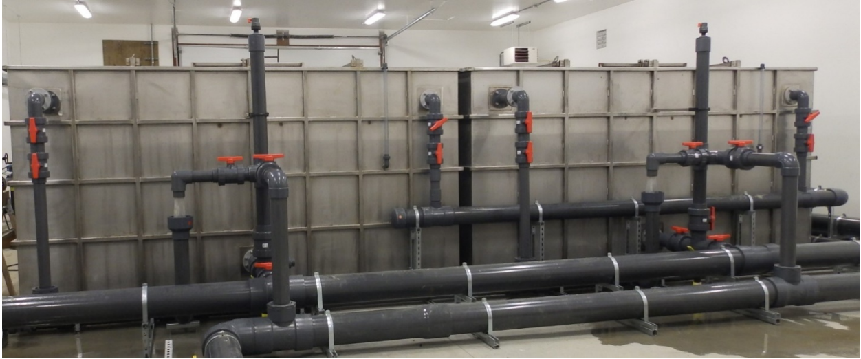
Front of filters #1 and #2
