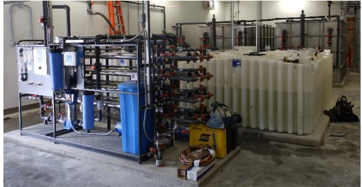
**Filtered water pumped into nano-filtration system**
