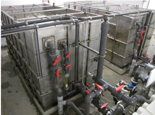
**Filters producing to storage tank**
