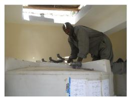
Constructing and installing the MEL filter components.
