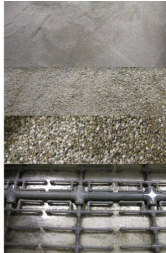
Figure 2. Photos of actual drainage pipes and underdrain layers.
