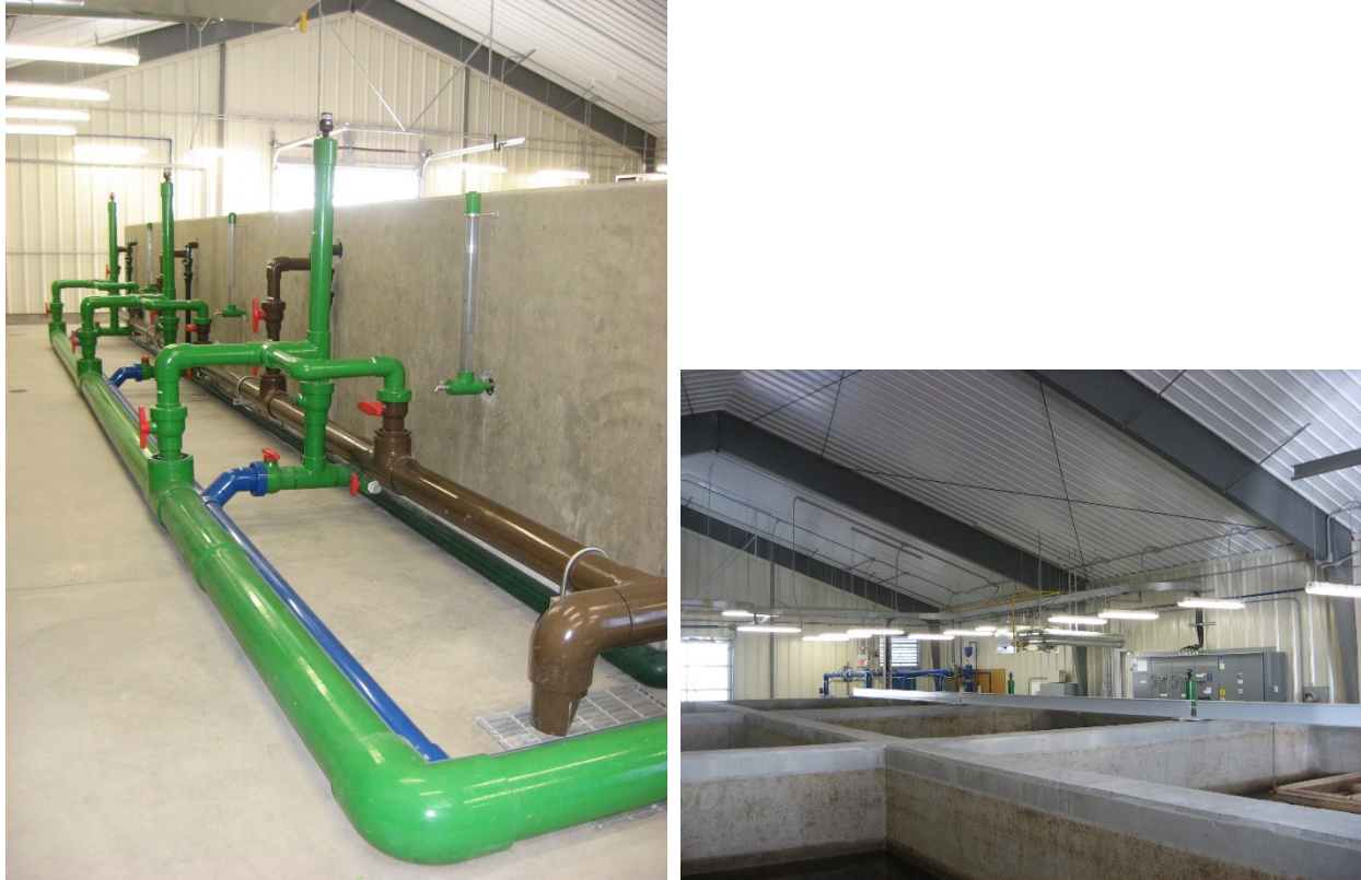
Figure 18. Photos of cluster of six 4m x 4m x 2m cast-in-place MEL type filters.
