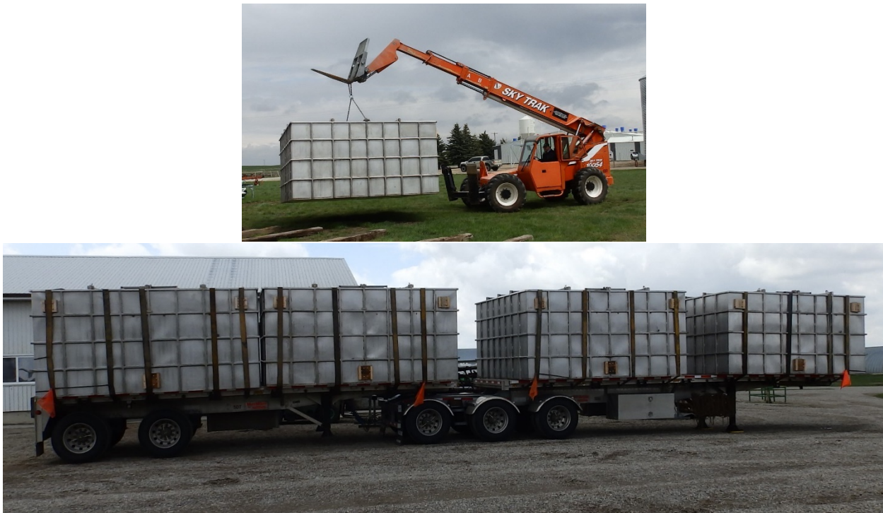
Figure 15. MEL 4m x 4m x 2m filter being loaded and transported.
