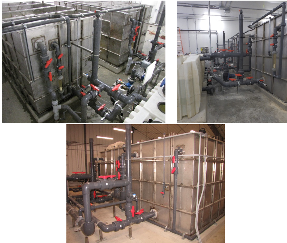
Figure 16. Photos of MEL 2m x 4m x 2m filter installations.
