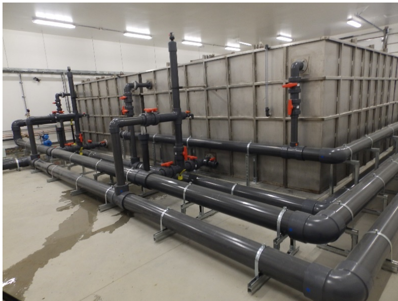
Figure 17. Photo of MEL 4m x 4m x 2m filter installation.
