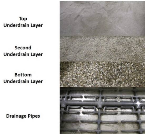
Figure 2. Photos of actual drainage pipes and underdrain layers.
