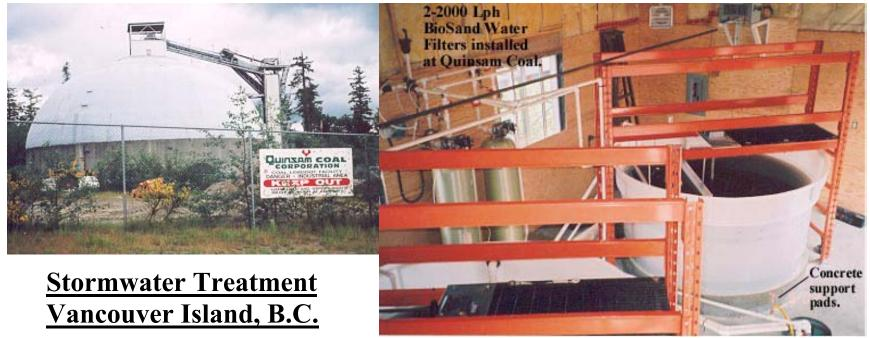
Stormwater runoff from coal loading pads must be treated prior to discharge into ocean. 2x2000 lph BioSand Filters
