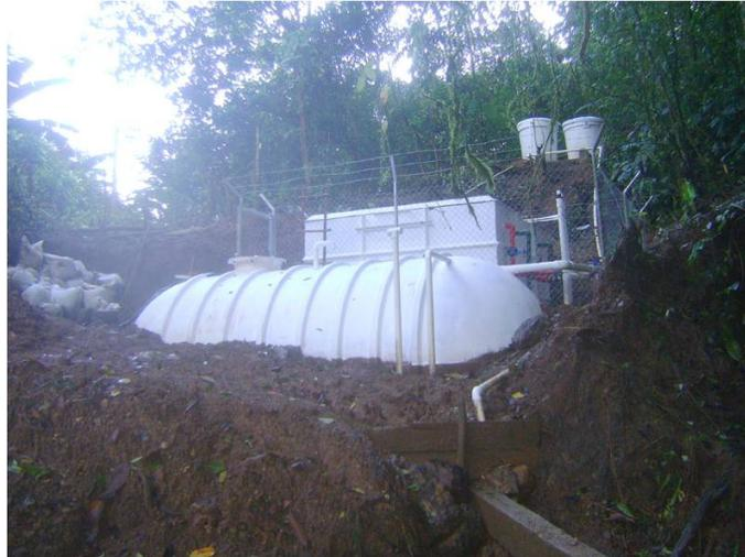
Figure 7. Photograph of Punta Huina water treatment plant showing treated water storage tank, filters and backwash tanks.
