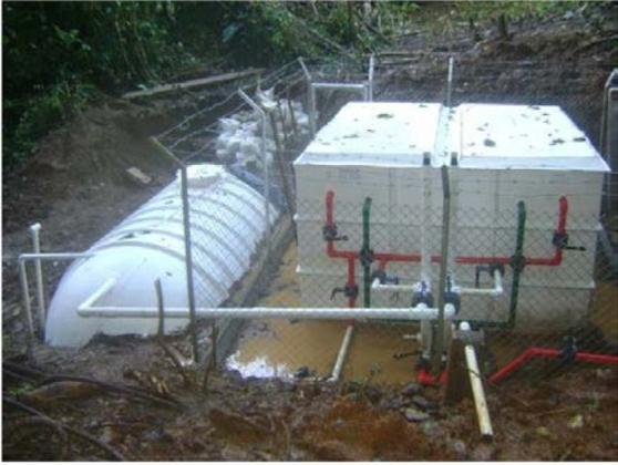
Figure 6. Photo of filters and treated water storage.
