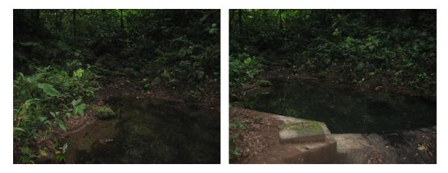
Figure 4. Stream where water is commanded by a small dam and coarse filter prior to transport to water treatment plant.
