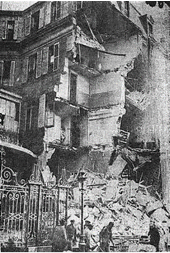
Damage from bombing
