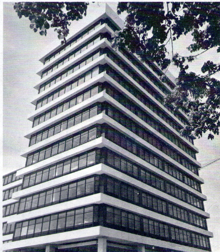
The towering Southampton headquarters of ACTS.
