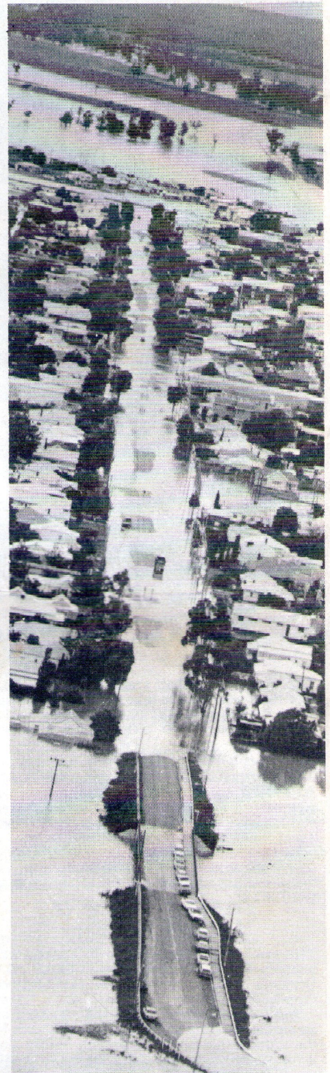
WATER Highway at the height of the Australian floods, with line of cars marooned on a bridge in the foreground.
