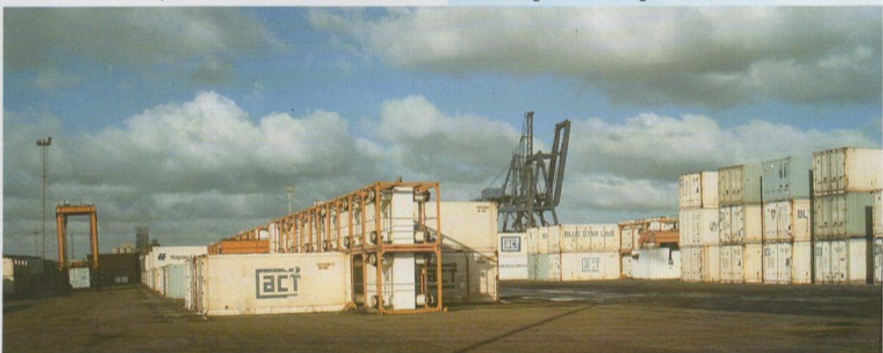
Partial view of the refrigerated stacking area at ACT(A)'s Northfleet Hope Terminal at Tilbury where the Unicore and Holima units can accommodate over 1,000 containers at one time. The new Data Logger System being installed will permit improved temperature surveillance, faster response times and even better cargo care for the 25,000 TEUs of refrigerated boxes handled per annum.
