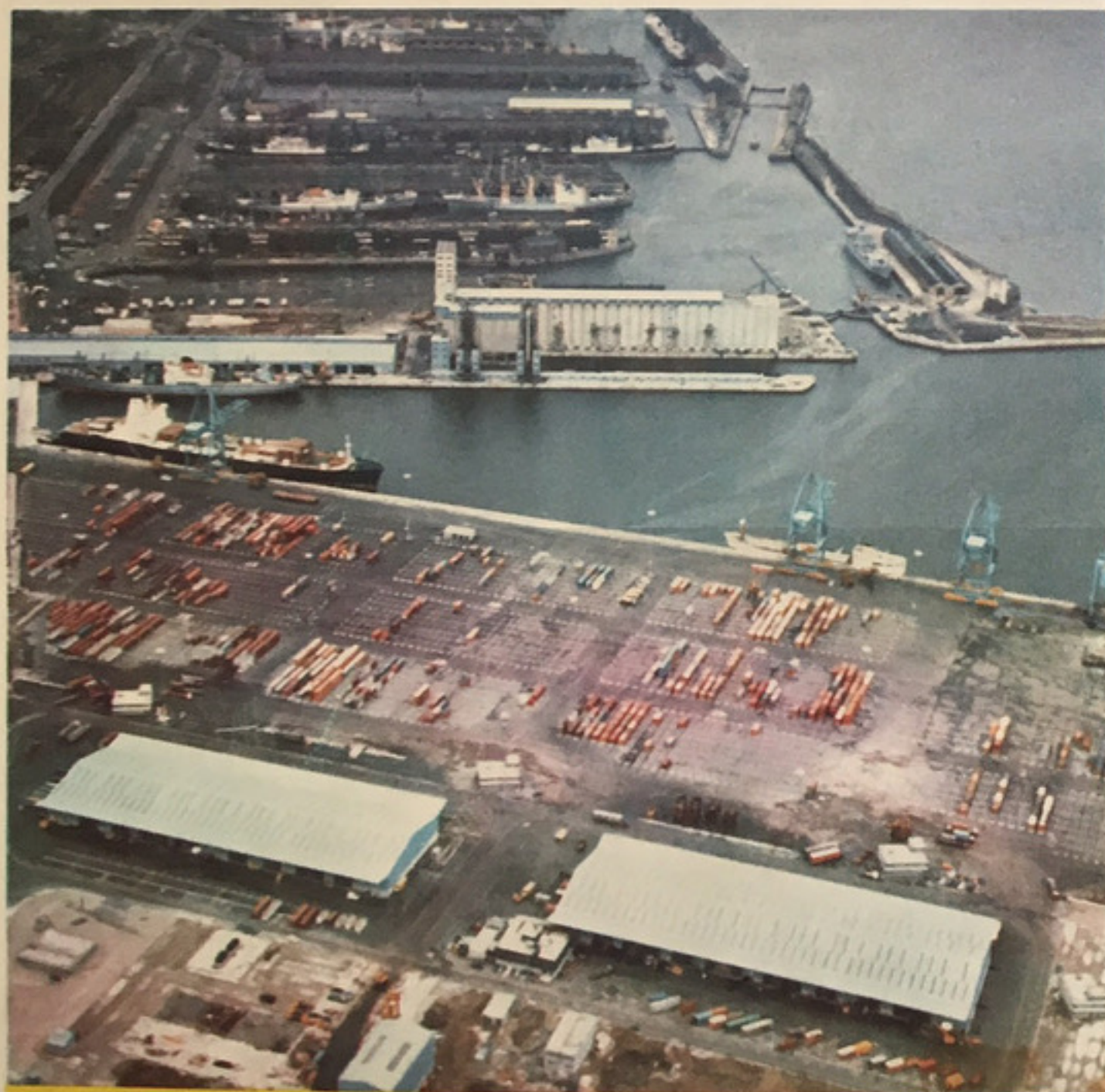
Right, an aerial view of Liverpool's new container port Seaforth showing the Grain terminal at left foreground and on the opposite side the giant container stacking area and 900-foot containership berth. Above, another view showing conventional cargo berths at centre background.
