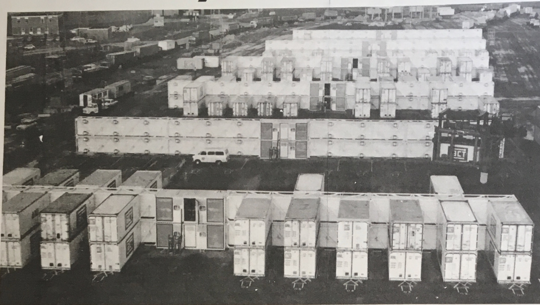
Bird's eye view of ACTA/ANL's 'Holima' refrigeration system at Tilbury. 'Reefers' are moved into position by straddle-carrier and stacked in double tiers. Each of the 12 units can be detached and re-assembled on a new site within 72 hours.
