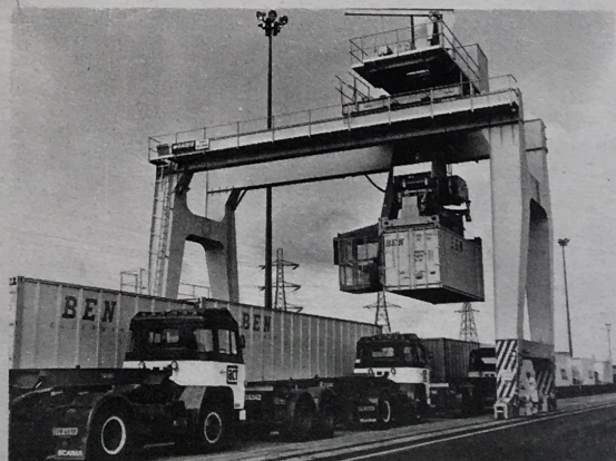
The container is lifted gently onto the train by this modern piece of loading machinery. More than 500,000 containers a year are carried by Freightliner service in Great Britain from their 24 terminals and six customs depots exclusively for export/import traffic.
