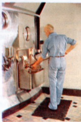
At the refinery the sugar is boiled in these large vacuum pans, each one holding 60 tons of granulated sugar.
