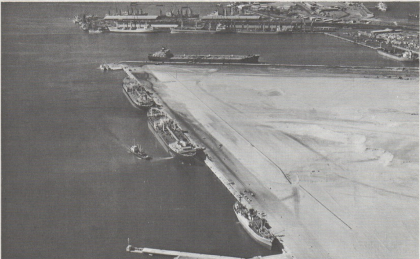
Partial view of the area where the new Durban container port will be located. It is presently under construction and scheduled for completion by mid-1977.
