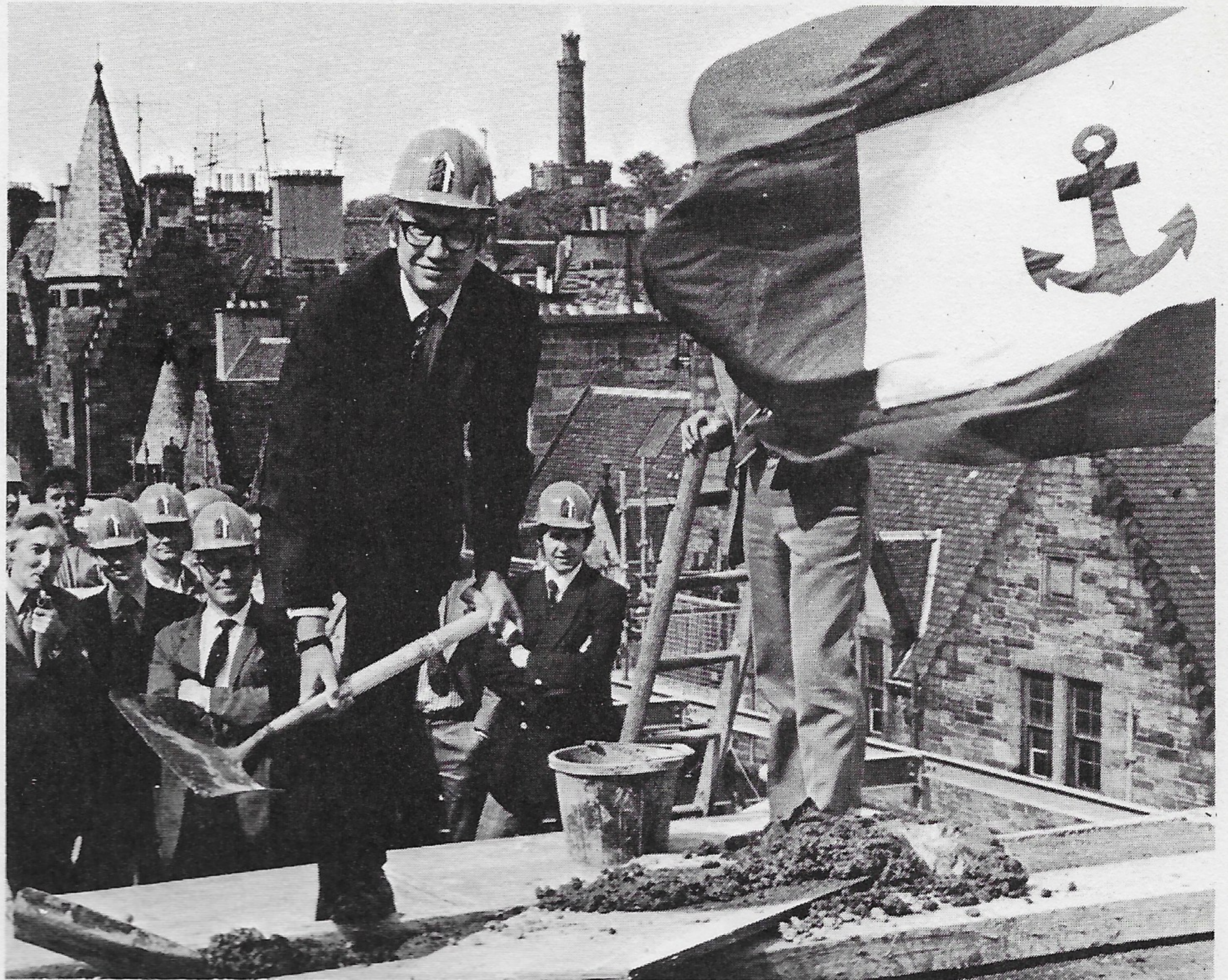
Mr. William Thomson, Joint Managing Director of Ben Line, helped lay the final structural concrete during a topping-out ceremony for the new Head Office of the Ben Line Group of Companies. The new six-storey building, which is expected to be ready by April 1977, occupies the complete length of the west side of St. Mary's Street in Edinburgh, just off the Royal Mile, the medieval thoroughfare which links the Castle with the Palace of Holyroodhouse.
